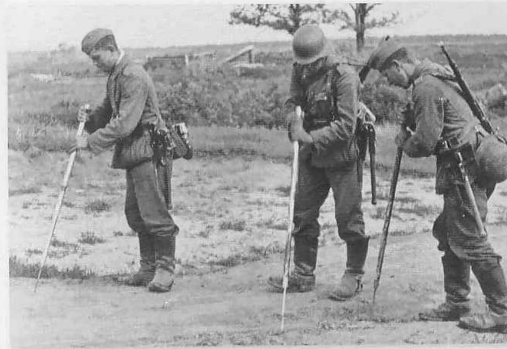
A German minesweeping team uses probes to search for Soviet mines on a dirt road. The Soviet defenders at Sevastopol used both TMD 40 anti-tank mines and PMD-6 anti-personnel mines. Each corps was clearing over 1,000 mines per day and was forced to use Tatar 'volunteers' and some Soviet POWs for mine clearance. (Nik Cornish Archive, WH544)
