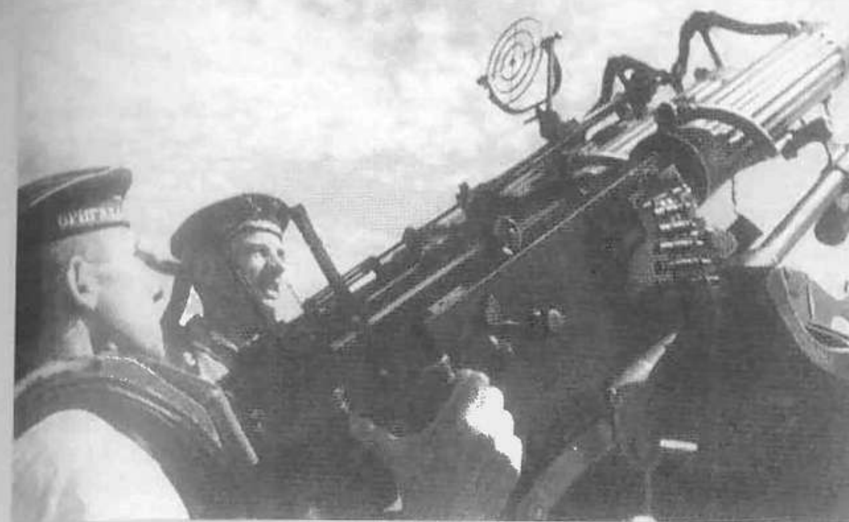
The Soviet Black Sea Fleet had one battalion with 18 Maxim quadruple 7.62mm anti-aircraft machine guns for air defence. This weapon was too short ranged and could only provide limited protection for some of the coastal batteries. (Author's collection)
